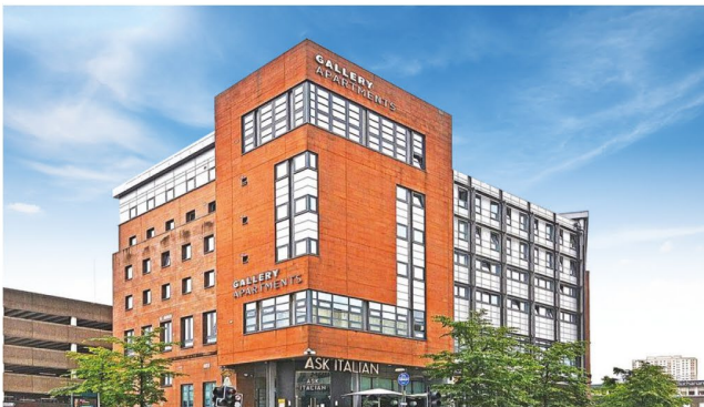
Gallery Apartments, Glasgow, UK
